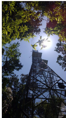
The Sentinel Phenocam is installed on TERN's flux monitoring infrastructure in the Daintree Rainforest in Queensland.
